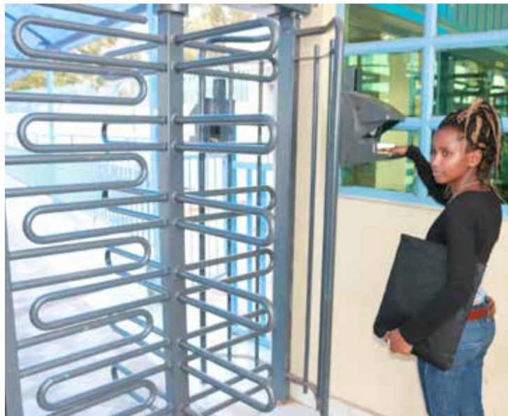
Biometric Access Control at Mount Kenya University -Thika Main Campus. MKU has complied with the Ministry of Education's directive that all universities capture student biometric data, becoming the first university to do so.
