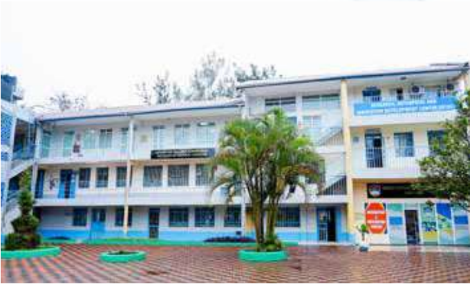
Research and Innovation facilities, Housing the Innovation Hub, Malaria Research Centre and the university Research centre.
