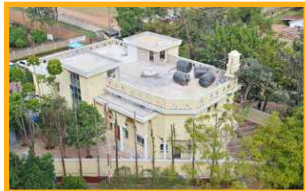
Expansion of Mount Kenya University Mosque, Main campus Thika.
