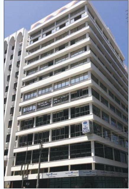
MKU Towers along Nkrumah Road, Mombasa County.
