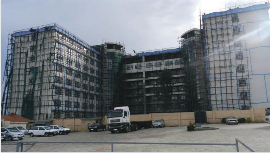
MKU Plaza in Nakuru town, at the final construction stage.
