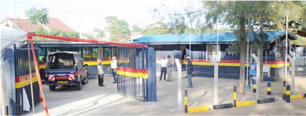
The newly commissioned police patrol base
